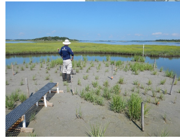
Dredged sediment added to ponded areas in fragmented marsh, Spartina planted
